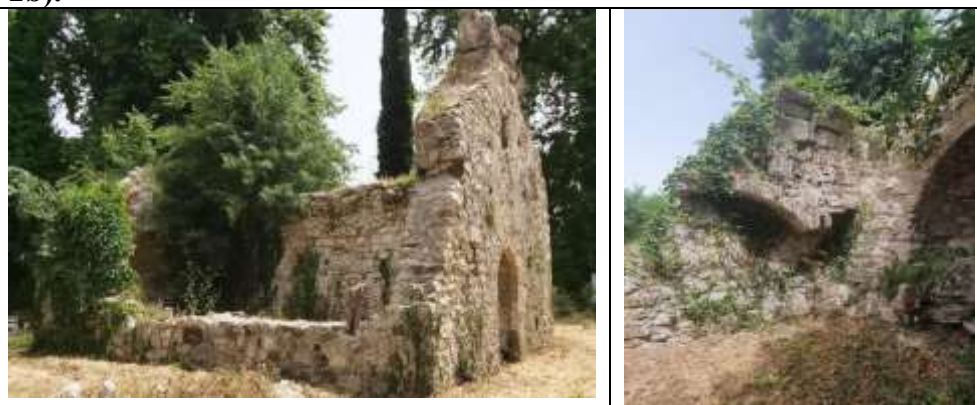
Figure 2: a- Church of St. Stephen, Blinisht, b- Fragments of fresco traces inside the church. (Source: The Author 2021)
